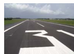
Runway 13-31 after Construction
